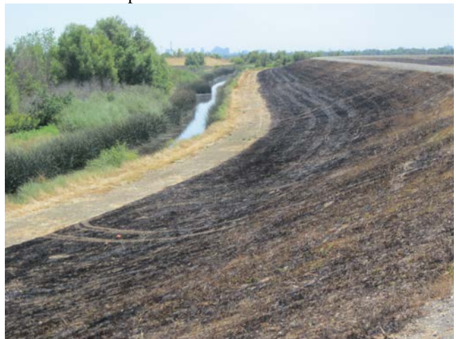
Photo 12. View toward channel in Willow Slough Bypass. The BSA is out of view on right, beyond levee. 11 June 2015.
