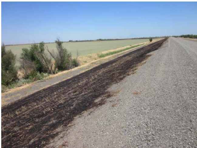
Photo 5. View northwest from atop the Yolo Bypass levee (recently burned). A few willows ( Salix spp.) occur in a dry ditch on far left. 11 June 2015.
